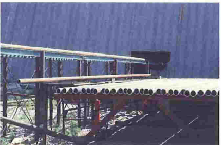
Manufacturing: The automated system for feeding cut pipe to the pipe bender. They red rams underneath lift the pipes up to the feed system.
