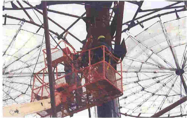
Installing the dual-axis tracking system.
