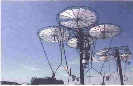
Field Testing: The original design had multiple solar towers in series connected driving a single turbine on the ground. In an effort to drive down construction costs a turbine was mounted directly to a single tower for use by only that tower.
