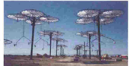
Installation: Our R&D towers being converted to commercial spec units.
