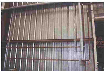
Early Manufacturing: The walls had to be outfitted with welding stations along with electrical and compressed air outlets.
