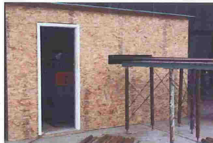
Manufacturing: Installed pipe-bender with insulated housing.
