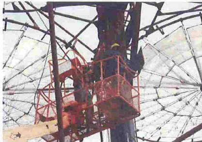
Manufacturing: Jeremy installing the new and final ram for the dual-axis solar tracking system.
