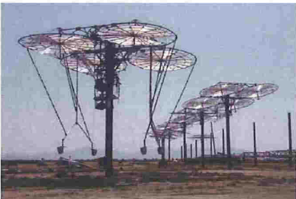
Installation: Starting to add the heat concentrators.
