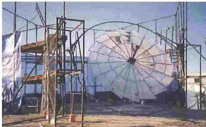
Second Tower Design: A two-disc solar tower concept was constructed with idea of lowering construction costs over the single-disc concept.
