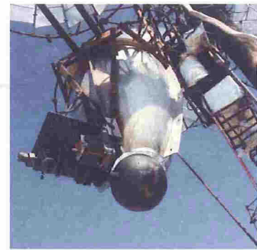
Installation: Close up of the newly installed gear-driven heat collectors or "magic ball".
