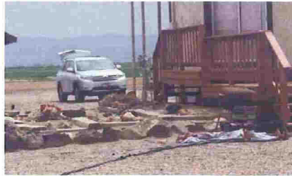
Installation: This shows the electrical cable that runs from the solar site to the grid home.
