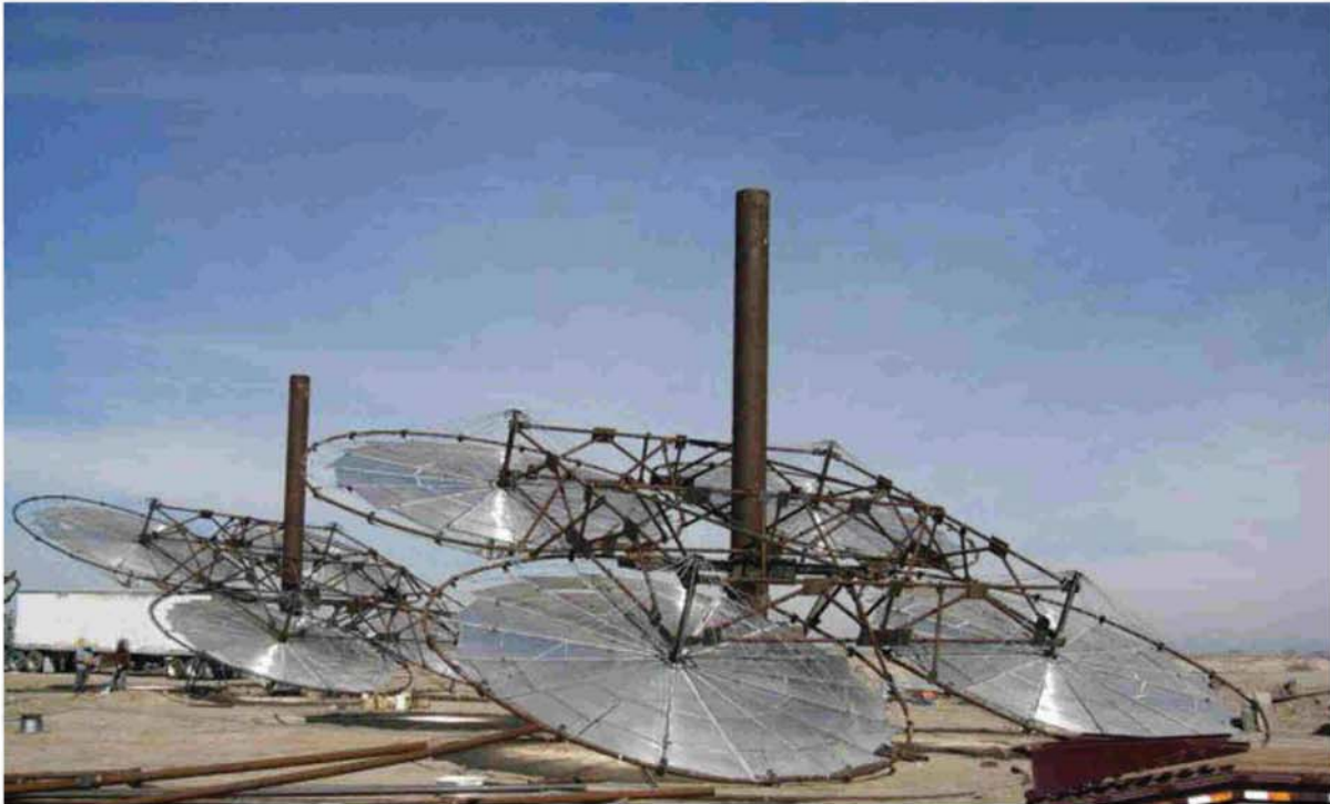
(Figure 6: IAUS solar field under construction)
